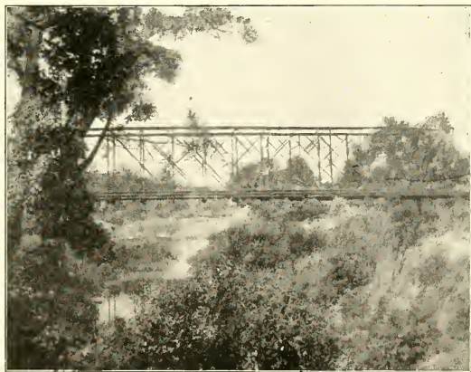
MODERN BRIDGES AT BLUFFTON
